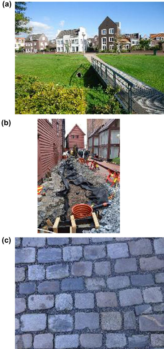
FIGURE 1 SUDS applied in areas with cultural deposits: swales in Leidse Rijn area (a), filter drains (b) and permeable pavement (c) implemented to preserve the cultural heritage site in Bergen (Norway).
